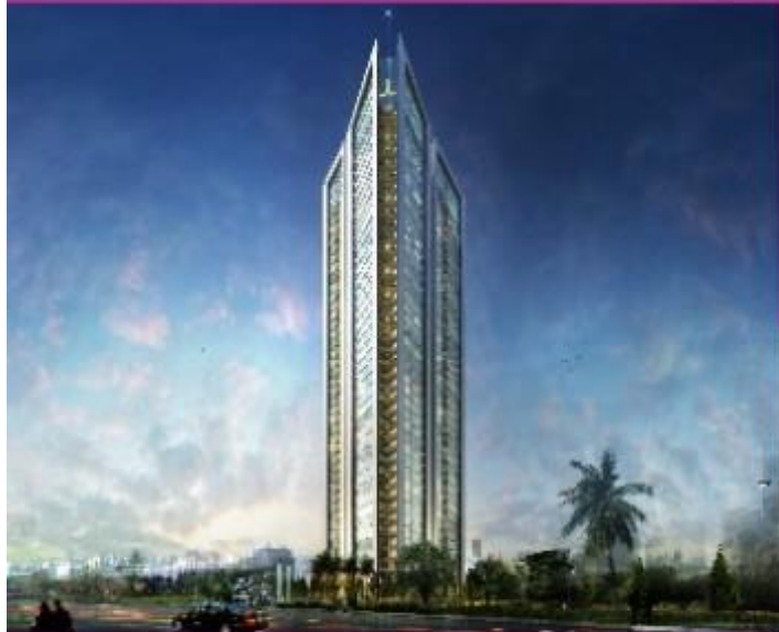
WESTLINE SIGNATURE NH66, NANTHOOR JUNCTION MANGALORE
